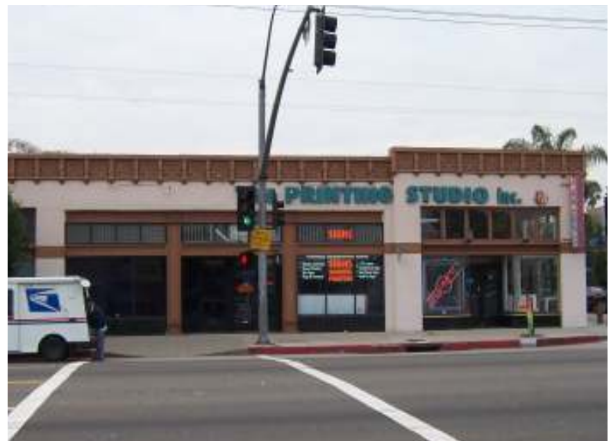
Guideline 23 Examples. These structures, built in the late 1920's, contain a variety of features that contribute to pedestrian-oriented design, including variations in material and façade planes, large windows, small-scale decorative elements, and street-edge definition.
