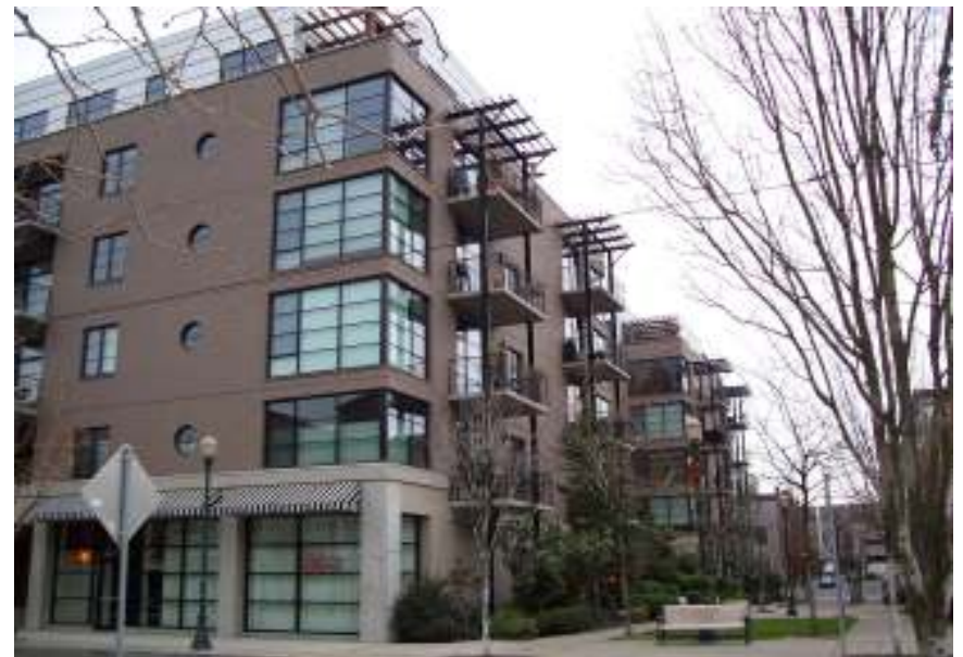
Guideline 4 Examples. Multi-story buildings shall employ subtle three-dimensional variations in massing to allow a break in the building envelope and provide visual interest.
