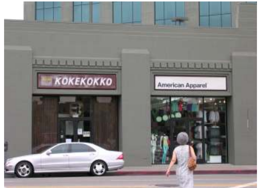
Standard 3b Example. These recessed storefront bays provide visual interest to pedestrians and help to break up the horizontality of an otherwise low-rise building.
