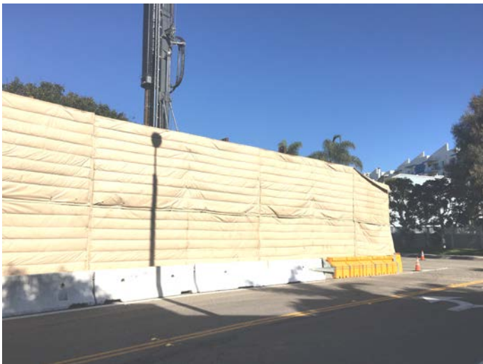
Example of Project Work Site: Sound Walls with K-Rail
